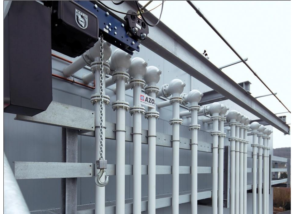
Special design of pipe bends for wear reduction
