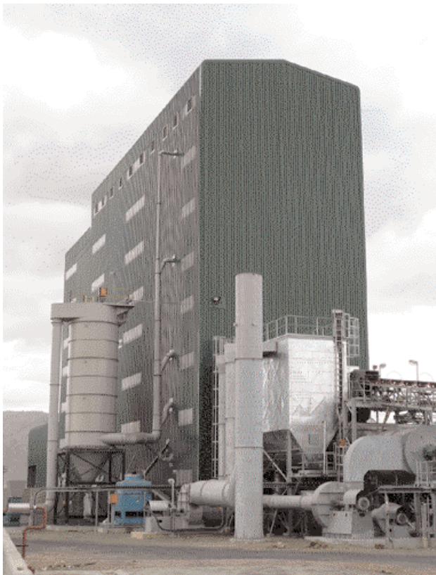
The seven storey building housing the dry separation plant with the sand drying and baghouse in foreground
